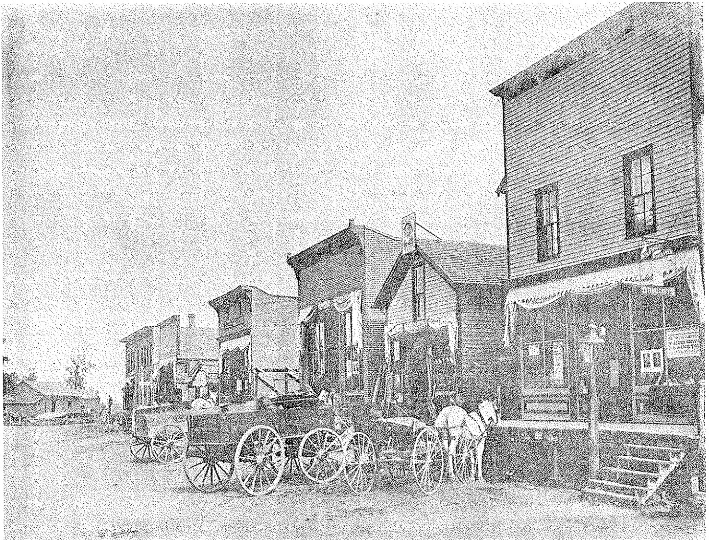
About 1888 r-l-Water Street - (note wooden side walks) Wolfinger and Gilligan Drug Store, Post Office in rear, Dr. Leightons office up stairs, Andrew Bee Tin Shop, Watkins Store, Bank, Orrie Gordon (dry goods), Dendel store, Millinery Shop(at one time a printer shop) the Hopkins Hotel and a mill that burned later.
