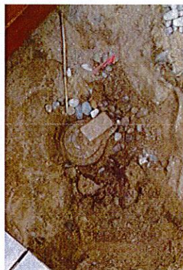
1.25" well (with jet pump) Buried Wellhead
